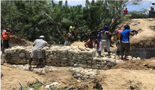
A program that helps control the erosion in Haiti. These Gabions filled with rocks placed by the roadside protects the only road that leads to the village of Brely.
